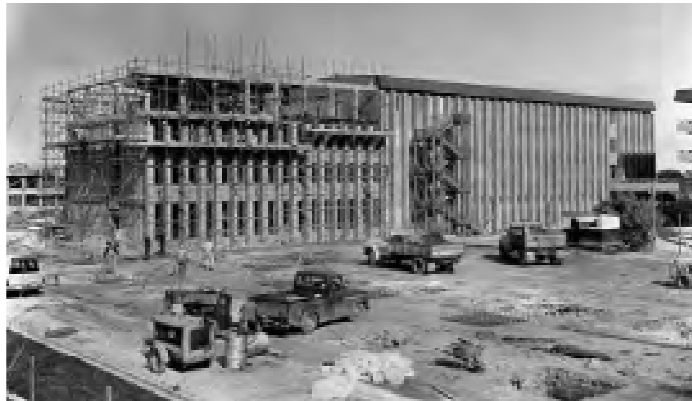
The construction of the Physics Building.
