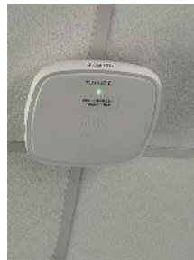
(Diagram 7.1.1 Image approved access point ceiling installation)
