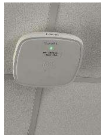
(Diagram 7.1.1 Image approved access point ceiling installation)
