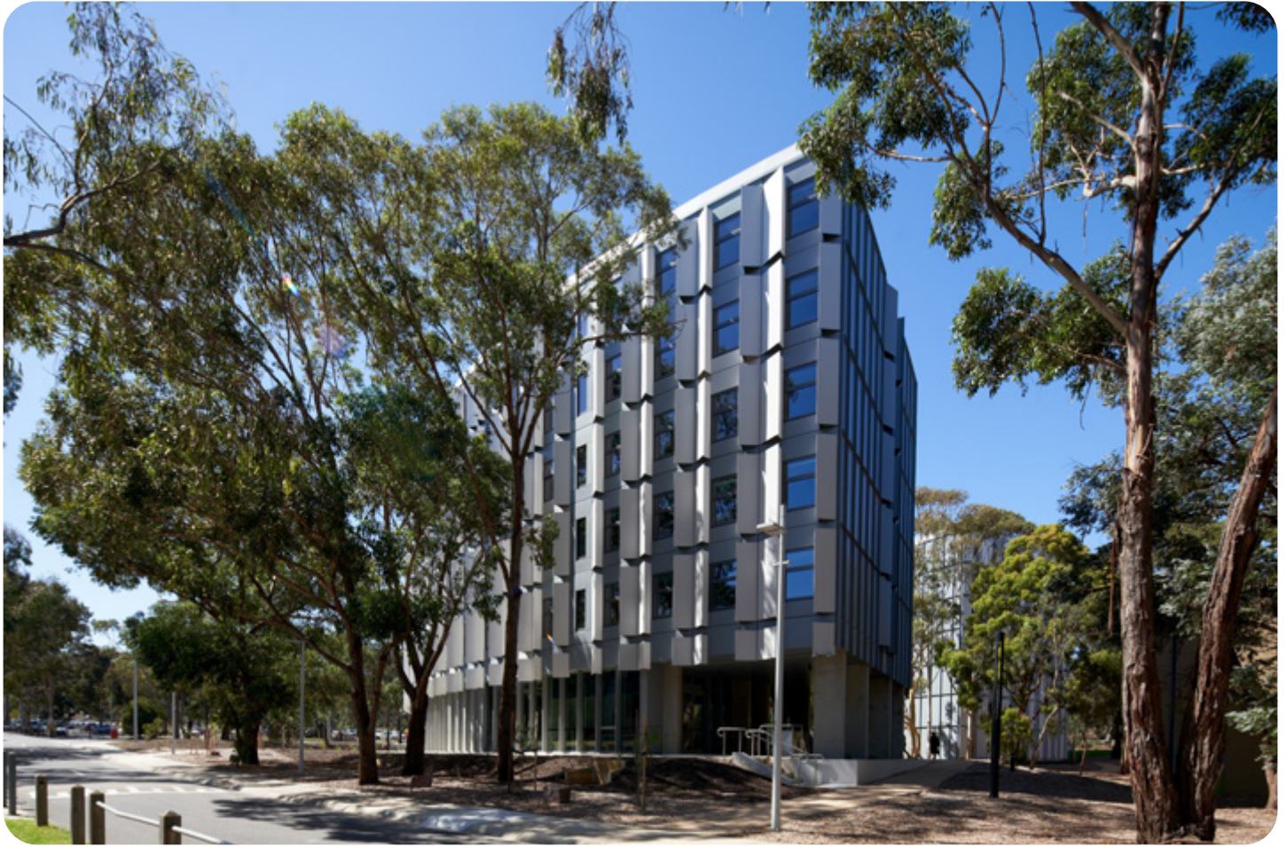
Above: State-of-the-art, 624-bed student accommodation with cross-laminated timber construction.
