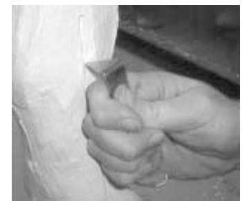
Figure 4. Plaster grooving using this simple tool.
