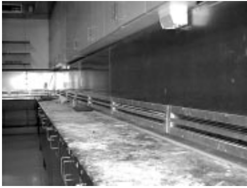
Figure 1. Bench extraction system.
