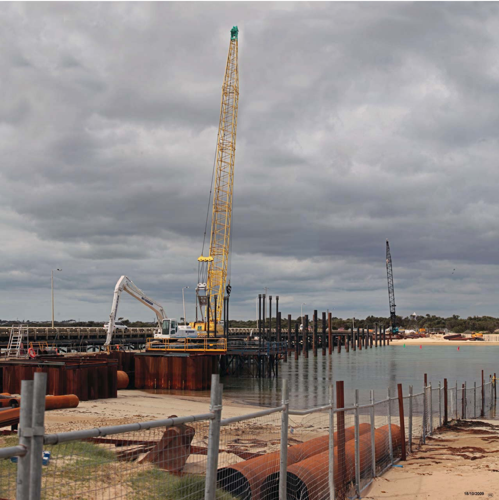
Stage 1 of bridge construction: Building temporary bridge and pedestrian bridge coffer dams
