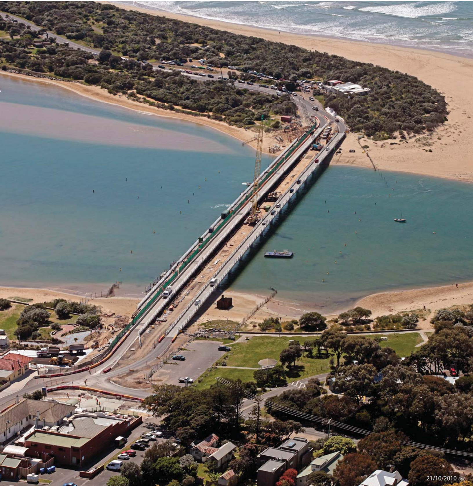
Stage 3 of bridge construction - Building Northern side of Road Bridge with Barwon Heads bound traffic on the newly constructed pedestrian bridge and Ocean Grove bound traffic on the newly constructed Southern side of the new road bridge.
